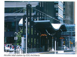
Nicollet Mall station by ESG Architects
