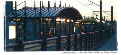
Franklin Avenue station by Barbour LaDouceur Design Group
