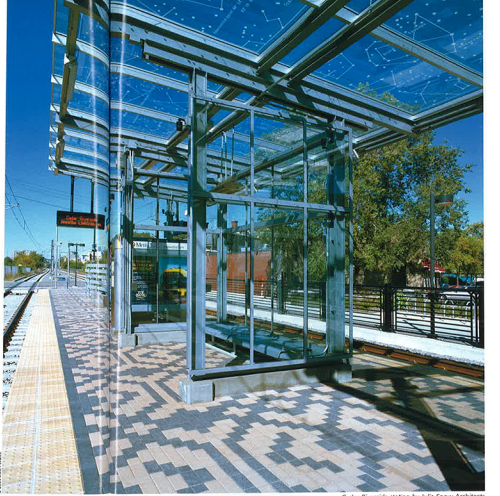
Cedar-Riverside station by Julie Snow Architects
